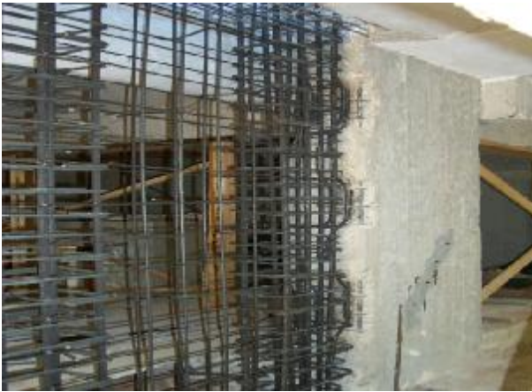
Figure 6 – Additional of RC shear wall to existing column
