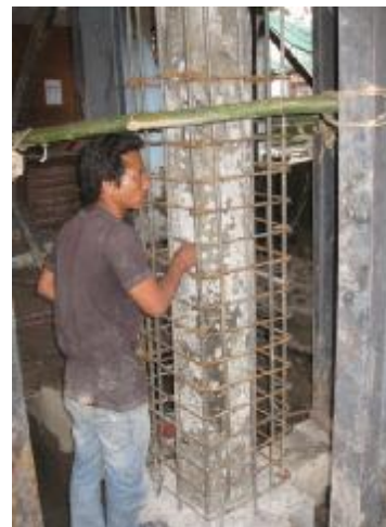
Figure 4 – Reinforcement of column and anchoring bars
