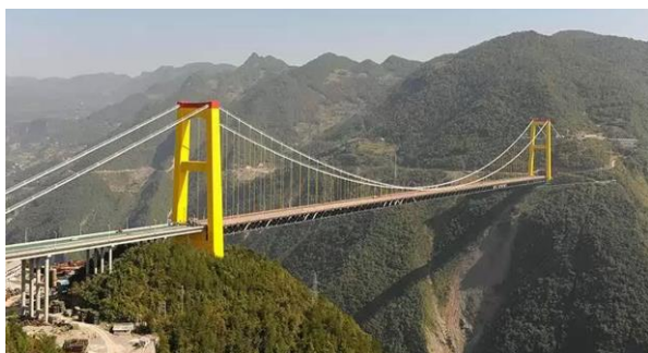
Figure 32 - Siduhe River Bridge, 2009. The length of the main span is 900 m, the distance the road from the bottom of the canyon is 496 m
