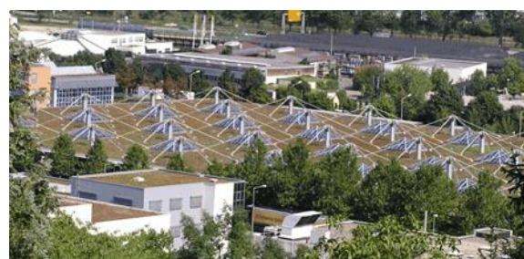
Figure 10 - Green roof Service LLC, Stuttgart, Germany (photo by G. Breuning)
