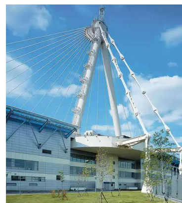
Figure 5 - The single pylon of the Ice Palace in Moscow, Russia
