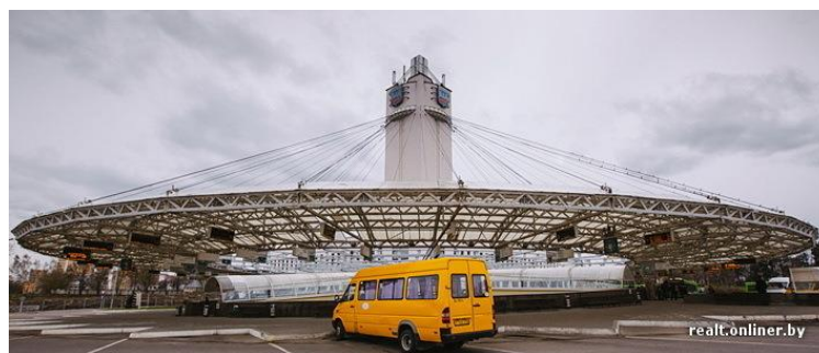
Figure 22 - The shed of a bus station in Minsk, Belorussia
