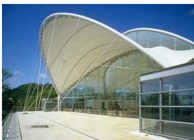
Figure 23 - Tent roof with stabilizing strands
