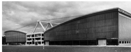
Figure 20 - A hangar at the airport of Frankfurt on the Main, Germany
