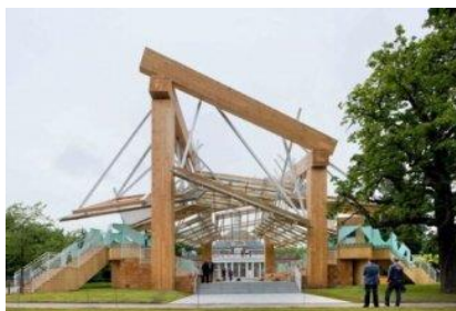
Figure 27 - Serpentine Gallery Pavilion, London, 2002
