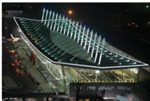
Figure 12 - A roof structure of railway station in Nanjing, Jiangsu Province, China
